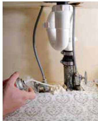
Spray foam seals gaps around pipes to prevent cold air from traveling up through those spaces, causing drafts and wasting energy.
