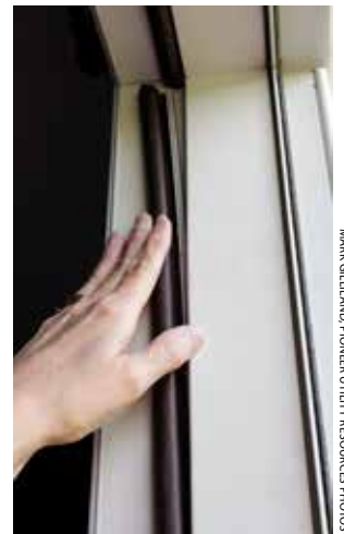
Weatherstripping helps seal drafts around exterior doors, which saves energy and improves comfort in your home.
