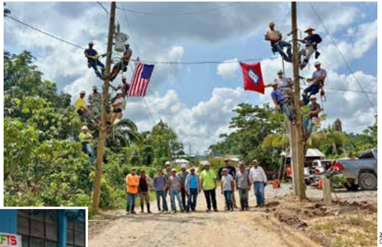
The Electric Cooperatives of Arkansas recently sent 16 lineworkers to assist a remote village in Guatemala.
