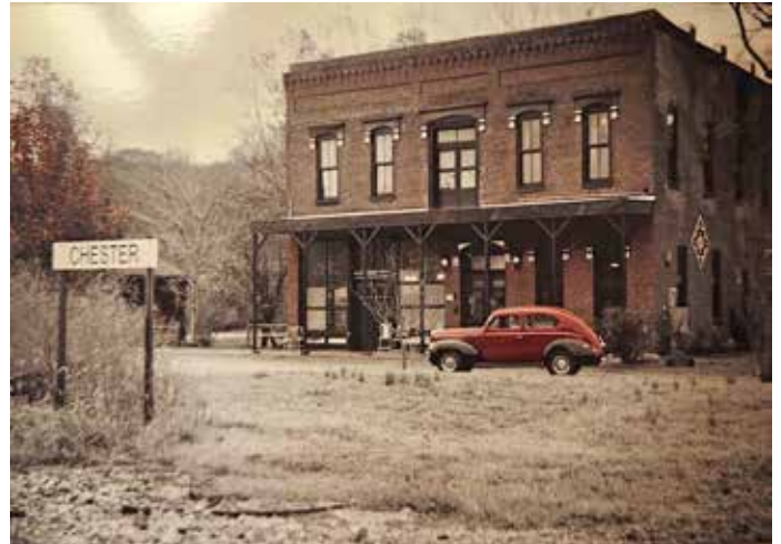
The historic Chester property that is now the Beard and Lady Inn, pictured here in a postcard, has undergone several makeovers.
