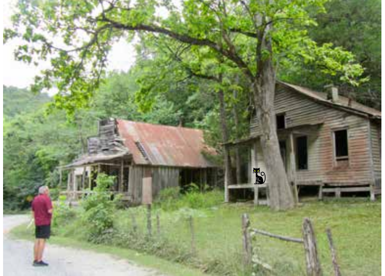
A visitor observes abandoned homes in Rush.
