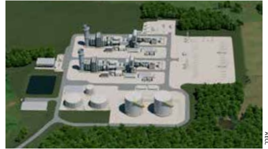
A rendering depicts AECC's future natural gas plant in Morris County, Texas, which will begin construction in 2026.
